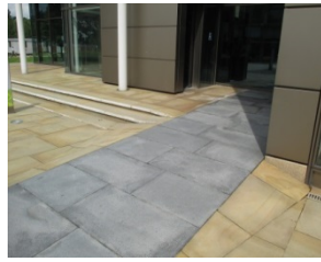
EBI main building ramp
