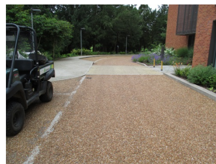
Access & parking at Mulberry Court.
